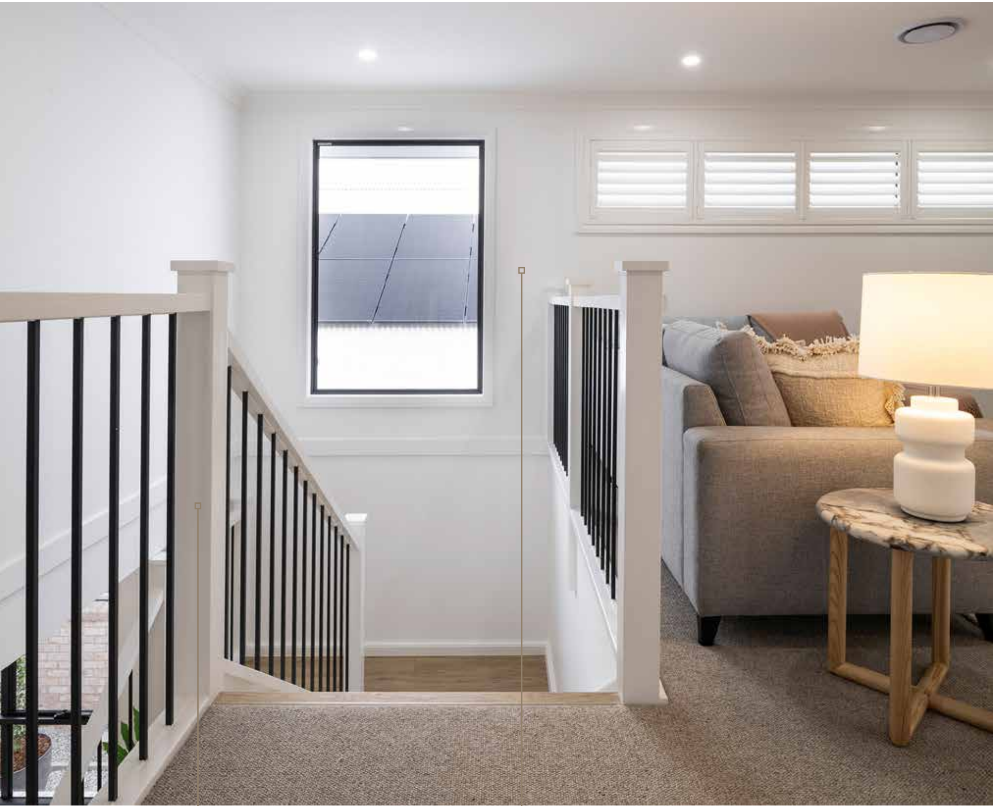
Custom made internal staircase including Pine stringers, posts, handrail with medium density fibreboard (MDF) treads/risers and choice of stainless steel or black 12x12mm metal balusters
