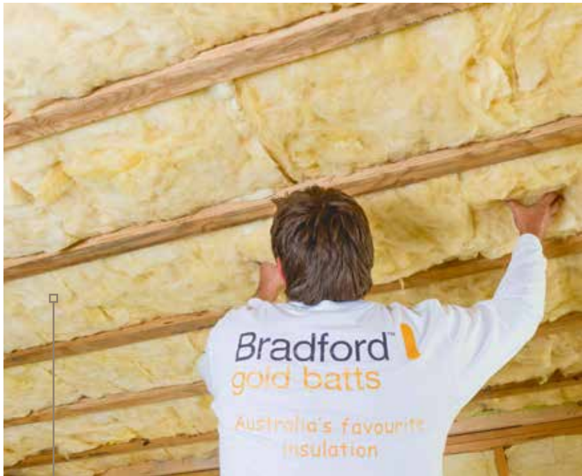
Bradford Gold Ceiling and Wall insulation (to comply with Basix requirements)
